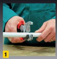
Cut the multi-calor (PE-X/AI/PE-X) or multi-eco (PE-X/AI/PE-HD) pipe with the shear creating a 90° angle with respect to the pipe axis
