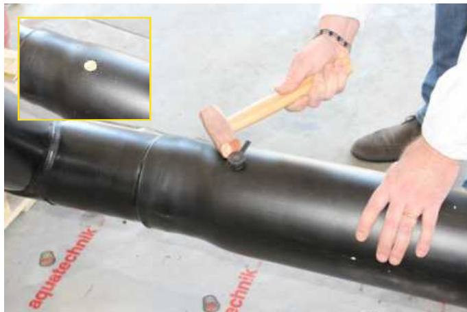
11 - With a light hammer blow, pop the drilled seasoning plugs. The hardened foam will look like the picture in the yellow box.
