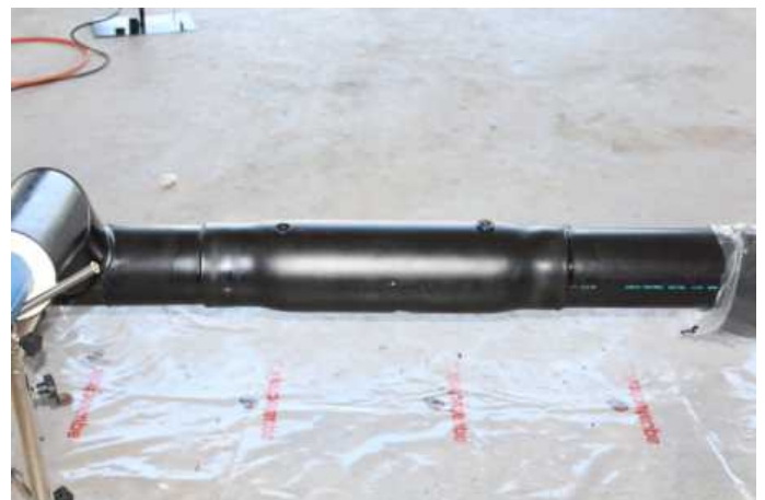
14 - Now, the installation of the single-seal restoration joint has been completed.
