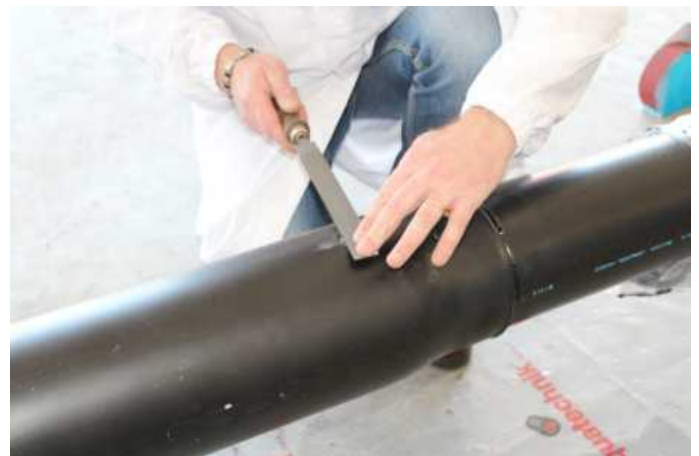
12 - With a rasp, slightly scrape the material to remove foam residues; after that, wipe with a cloth soaked in the cleaning liquid (item 50330) to finish the cleaning operation.
