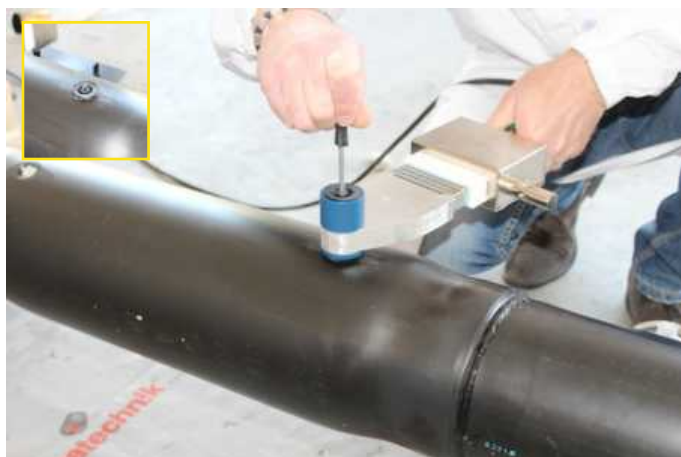
13 - Weld the supplied closing plugs by polyfusion, and then comply with melting and cooling times.
