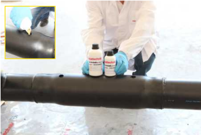
9 - Mix the bicomponent products by pouring the polyol content into the isocyanate container: after that, shake for maximum 2 seconds, and then pour the content into one of the two holes. WARNING! This operation must be carried out in very short times because the chemical reaction of the mixture is immediate
