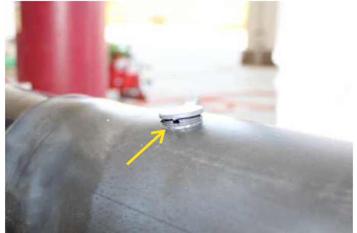
10 - Place the two supplied seasoning plugs by paying attention that the vent opening is not pushed inside the hole. After that, wait for about 20 minutes so that the introduced mixture becomes foam.
