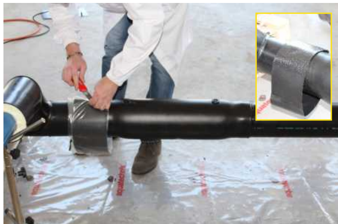
15 - After performing the cleaning operation with the cleaning liquid item 50330, remove the packaging film from the heat-shrinking band, and then place it on the casing pipe weld by paying attention that the middle line of the band correspond to the welding line.
